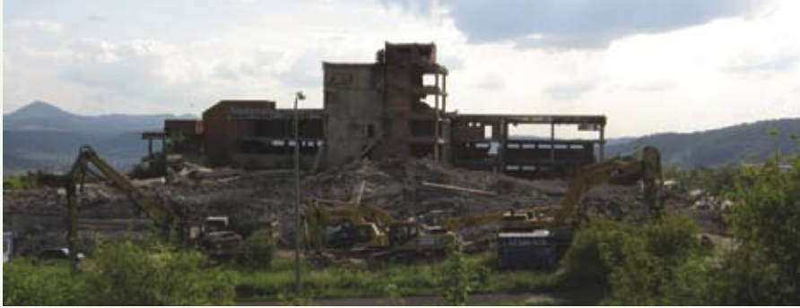
Demolition works in brownfield area
