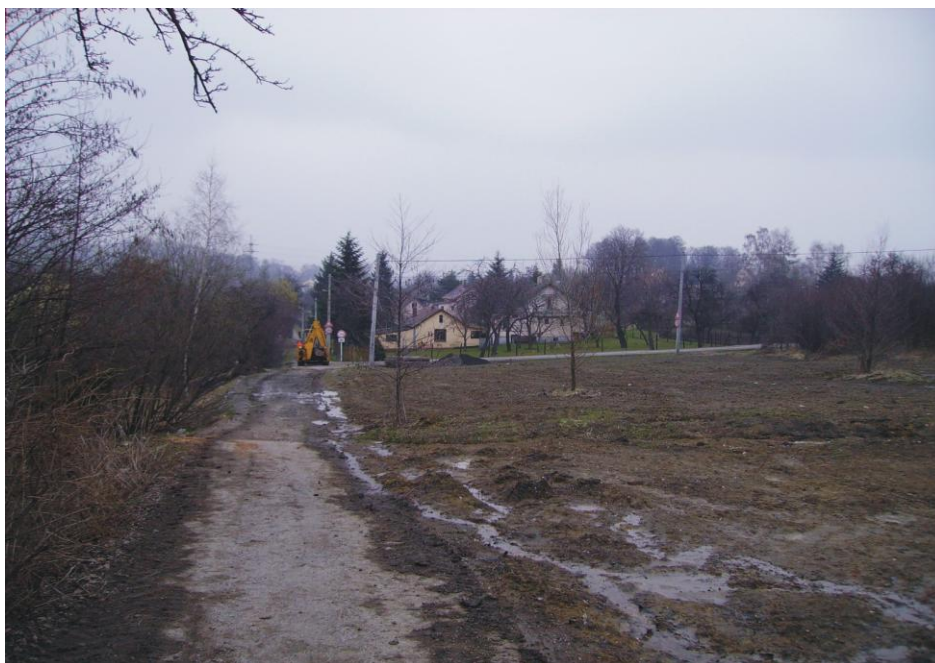
Figure 8. Executed ground shaping.
