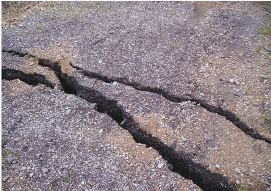
Figure 6. New cracks up to 10 cm wide and 90 cm deep.
