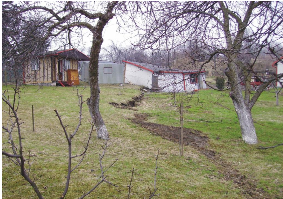
Figure 4. Recent movements on the side tear edge and a tilted tree.
