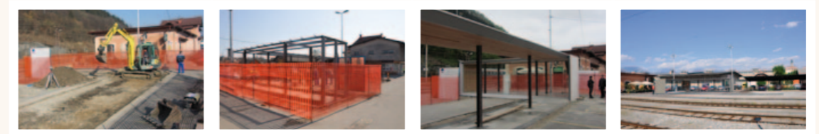
Fig. 22. Information point in four construction phases
