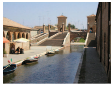
Fig. 25. Comacchio historical centre – Trepponti bridge
