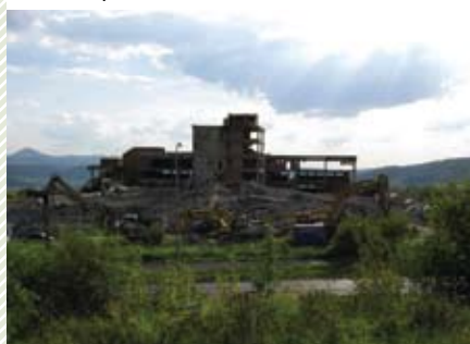
Demolition of a building in a degraded area
