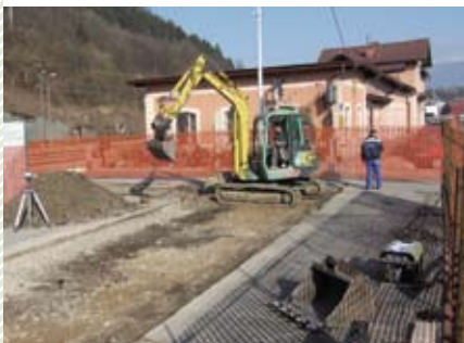
Construction works for the Info point
