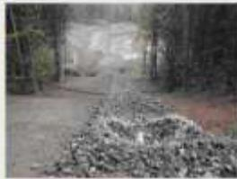
Constructed wetlands may include one or more ponds or compartments where AMD flows through preferably at a slow rate. The iron is oxidized and precipitated within the wetland. Acidity is neutralized by the vegetation photosynthesis and other biological activity which produces alkalinity.
