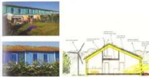
The 'Limmerland' passive houses are heated and cooled all year round without a separate heating distribution system using passive technologies. In winter, if necessary, each house can tap into the district heating system, when warm air is distributed by the ventilation system. Supplementary heating needs are around 15kWh per m<sup>2</sup>; a passive house consumes one-seventh of the heating energy of a conventional new house.
