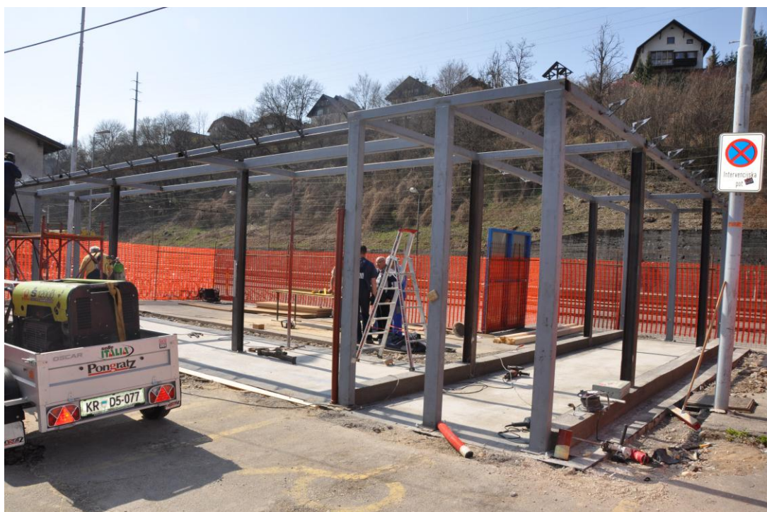
Construction on 22 nd of march 2012
