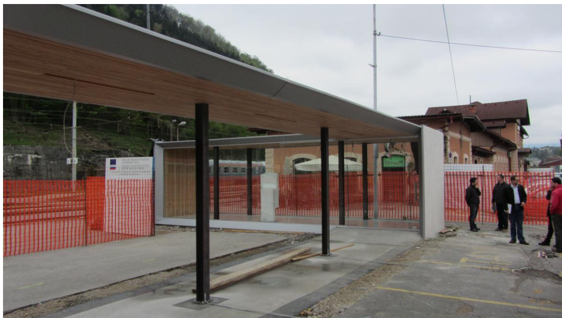
Construction on 23 rd april 2012
